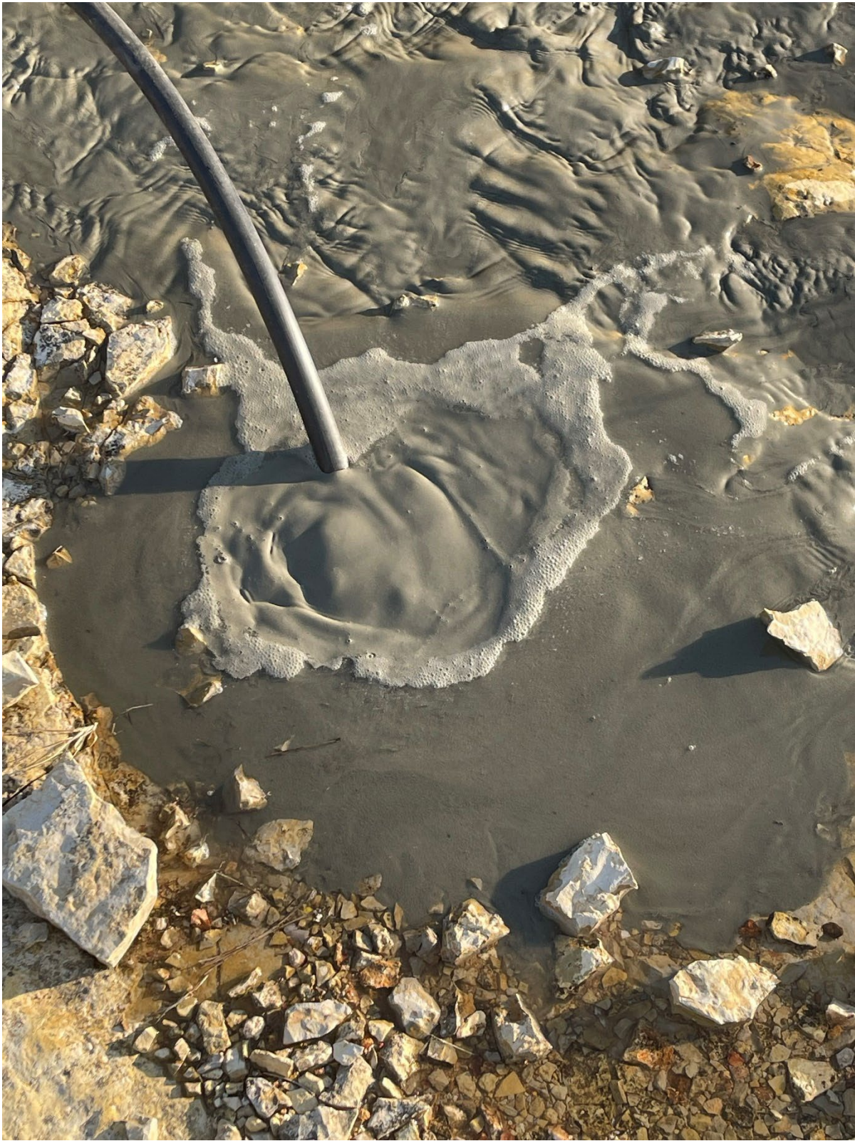
Placing concrete to ground surface in EB-1
